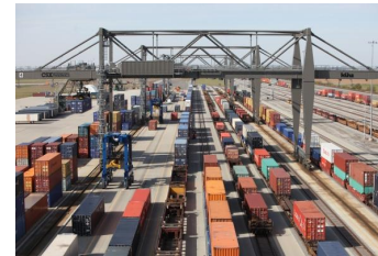
Inland Rail Terminal = CY Rail Ramp term
